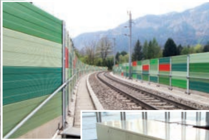
BETONYP® as noise reduction wall
