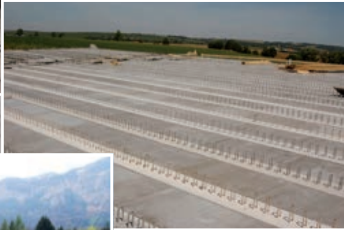
BETONYP® as formwork
